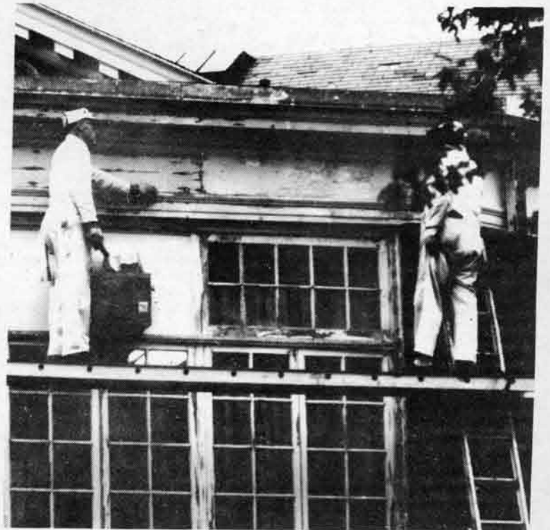
The long, slow, continuous job of painting the Administration building, begun last spring, neared completion this week as workmen scraped old paint from a section badly in need of a new coat.
